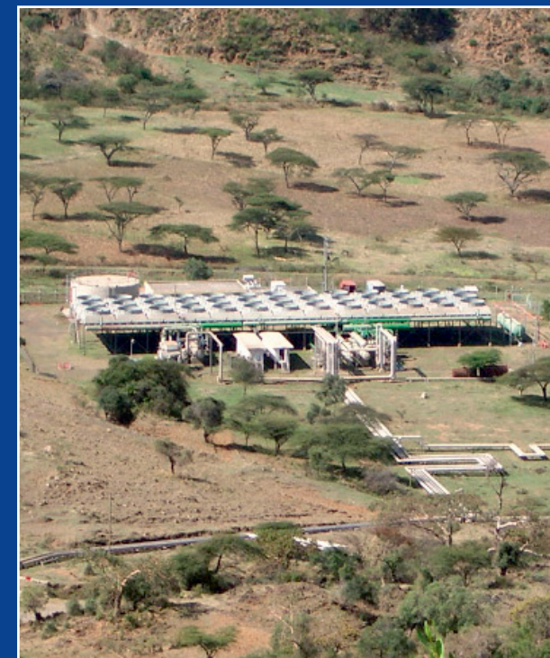
Aluto Langano Power Plant (8 MW), Ethiopia
